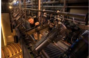
The investment extended to over 600 Vari-Lite SL Series and Strand fixtures. These include a broad array of the latest LED technology, from fixed PLPROFILE4 MKII white light ellipsoidals to color changing moving head fixtures, as well as conventional incandescent models. The end result is a beautifully designed, fully equipped and future-proofed creative facility, which is set to inspire future generations of performers and technicians.
