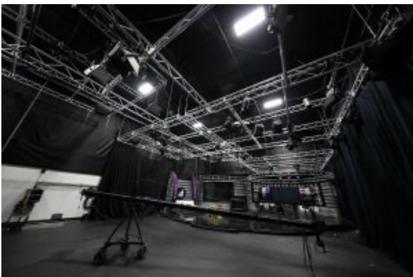
Trussing in studio one
