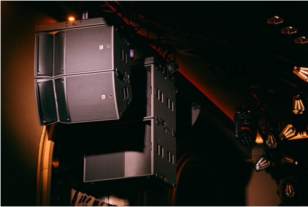
(Above): The main dance floor features two flown arrays of one A15 Wide and one A15 Focus with two KS21 subwoofers per side
