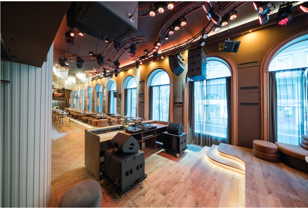
(Above): DJ monitoring is handled by groundstacks of two X12 atop two KS21 subwoofers
