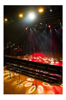
Robe makes up 90% of the lighting with eight Pointes, six LEDWash 1200s, eight LEDWash 800s, four ROBIN DLS Spots, eight MMX Spots and eight MMX WashBeams. All these fixtures are fitted with the Lumen Radio wireless DMX card.
