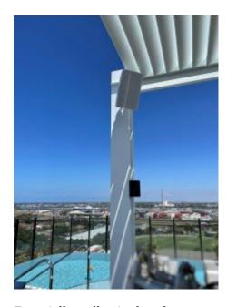
Especially well-suited to those spaces exposed to the elements, the MX801 features a sealed enclosure design and additional weather resistance connector covers (IPMX1), ensuring complete outdoor protection and enabling the loudspeaker system to be rated up to IP67. RKP Engineering chose to add the optional IPMX1 due to the system's roof location and close proximity to the venue's infinity pool.
