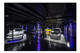
Björn Arnason's lighting design incorporates 42 x Robe PARFect S1s which he chose because they were "perfect" for the application. They are installed on a series of trusses in the roof.
