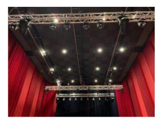
The brand-new Theater Zuidplein in Rotterdam, the Netherlands, has over 200 Robe LED fixtures – including T1 Profiles, Spiiders, LEDBeam 150s and ParFect 150s – installed as part of an all-LED lighting rig. It is among the first cultural centres worldwide to have no dimmers!
