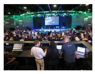
The installation sees circular trussing dead hung off the main structure of the roof. Longman FacePars serve as truss warmers and Longman F4Ups for the stage wash.
