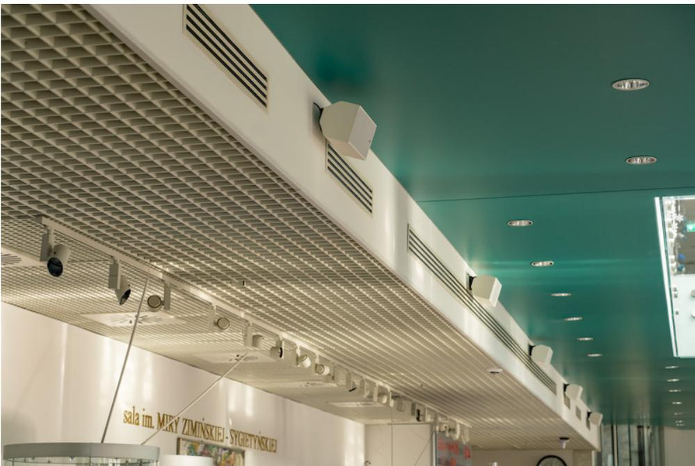
The lower lobby is equipped with eight L-Acoustics X6i wideband speakers and an SB10i W subwoofer
