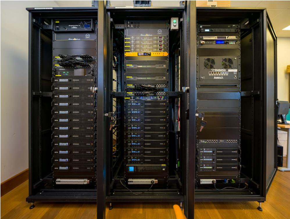
The system is powered by two L-ISA Processor II, two P1 processors, twelve LA7.16 and eight LA4X amplified controllers. Managed through a comprehensive Digico control system
