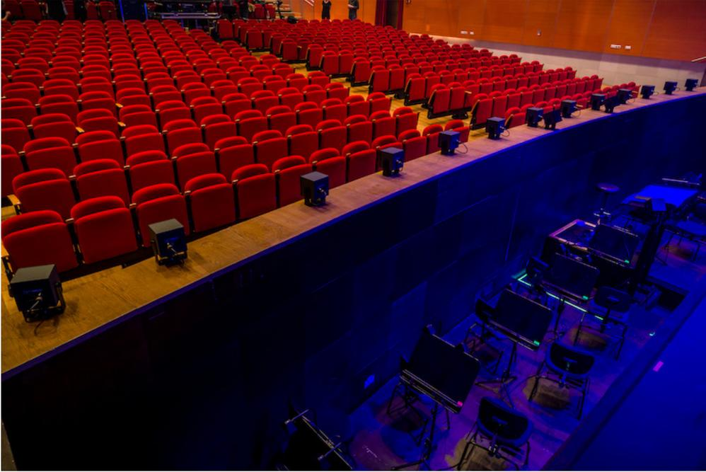
Fifteen L-Acoustics 5XT coaxial speakers are spread across the stage lip provide spatial in-fill
