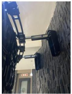
The Absen screen, structural support and screen border cladding was fixed to the wall with heavy duty telescopic slides. Each 500mm telescopic slide (five in total), has a safe working load of 440kg at full extension of 1m.
