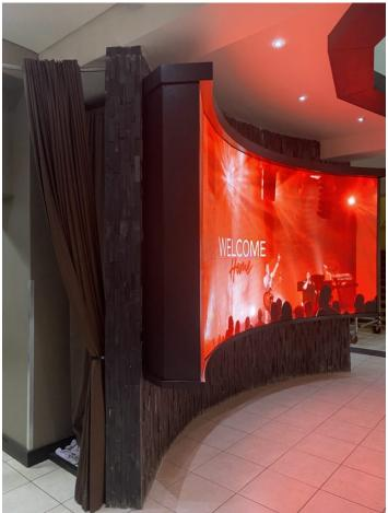
To provide an aesthetically pleasing appearance, DWR created a sheet metal cladded border around the entire Absen screen.
