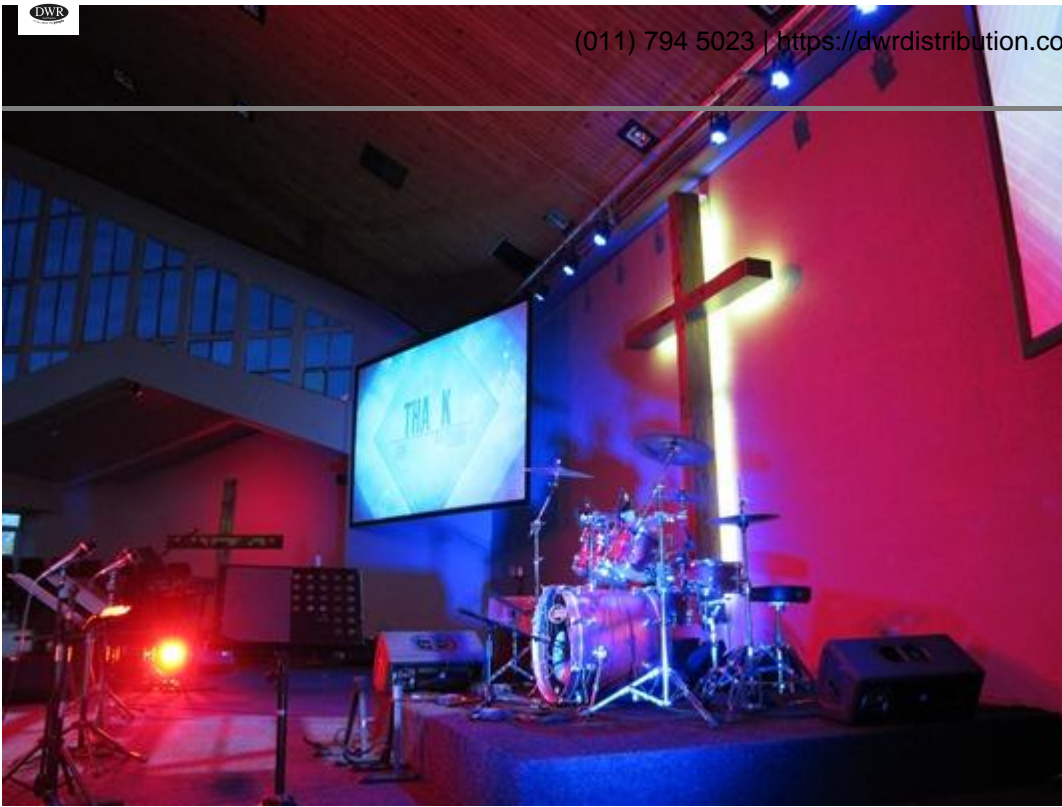
The lighting system now
