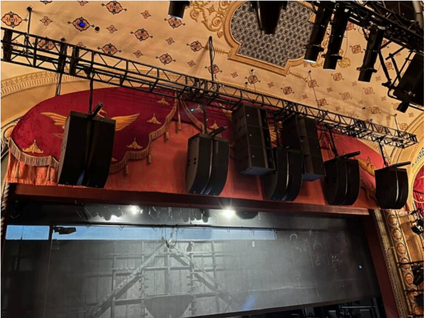
The Outsiders' frontal truss features Broadway's first deployment of L-Acoustics L Series arrays (photo credit: Cody Spencer)
