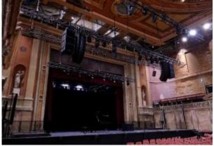
"L-Acoustics did the final tuning of the system, which is perfectly balanced for the room," Brookes continues. "There isn't the need for much EQ as we have the right placement and the right type of boxes. We have achieved complete coverage, with the main arrays pretty much doing the entire room, with six 5XT for lower SPL shows, or six X8 for louder shows, providing fill for the front few rows. This means there's no need for additional, confusing sources."
