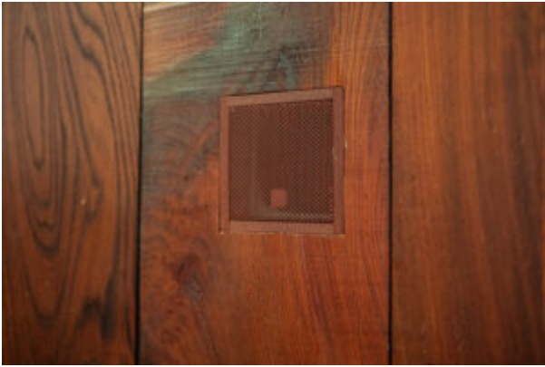
The L-Acoustics X4i installed inside the stage lip of the Nō Theatre.
