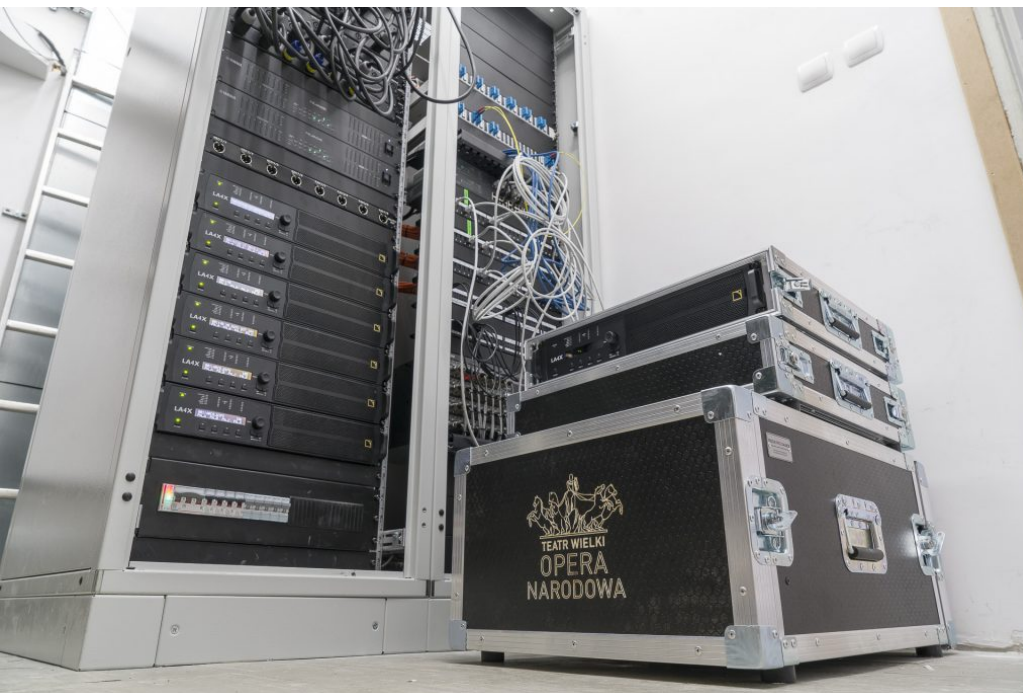
The entire system is powered using six L-Acoustics LA4X amplified controllers in fixed rack, with two LA4X in mobile racks available when needed.
