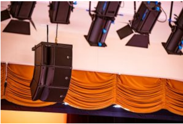
Close up of the centre cluster of L-Acoustics A10i Focus and A10i Wide.
