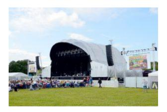
The Polygon roof systems comes in four different sizes and IPS will be showcasing the 18m. version at the Showman's Show. To convert from one size to the other, only some straight length parts need to be added, all corner parts remain the same. This solution minimizes the amount of parts needed and offers maximum flexibility.
