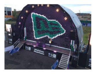
Apart from the width of the stage, also the depth can be varied. This makes the roof system adaptable to any type of event. After an initial test build in early June this year, IPS already has used this roof on several projects this summer, like the Tom Jones concert at Holkham Hall.
