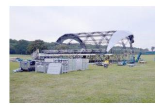
Based on H40V truss, the Polygon XII roof system offers a multi-functional and cost-effective solution. The straight truss lengths convert into a curved "tunnel" type roof with the addition of special corner sections.
