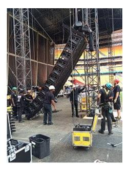
South Africa: When it comes to suspending line arrays for large-scale events, In-Harmony Productions rely on ProLyft motors from Prolyte. With six one Ton Prolyft motors in stock already, they recently made an investment of an additional two ton motor to keep up with demand.
