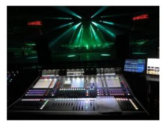
From an audio perspective, this show is huge. The FOH and monitor consoles – both DiGiCo SD7s – are maxed out, plus there is an SD11B deployed for the shout system.
