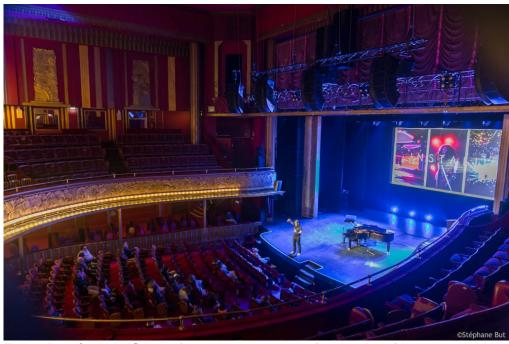
Folies Bergère's L-ISA configuration comprises five hangs of L-Acoustics A15 for the main system, with L-Acoustics X8 providing under balcony fill to perfectly cover the entire auditorium.
