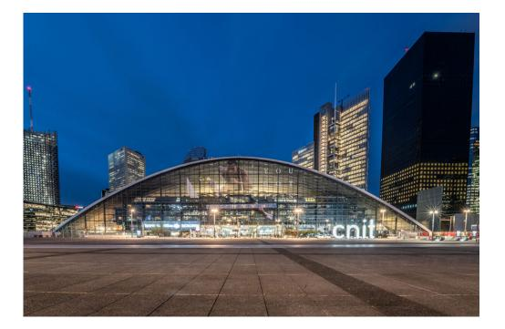
The imposing concrete 'vault' as it is known, is 46 metres high and each side is 218 meters long, forming part of an equilateral triangle. Three glass façades – with convex curves on two sides – each span 206 meters and allow daylight and sun to stream through into the space.
