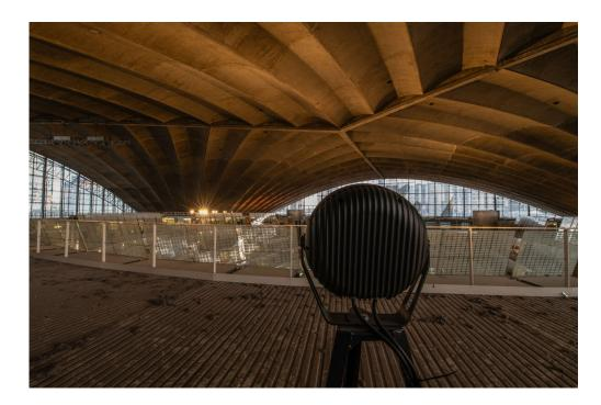
The 1.2-metre-high eye-level stands – in smart graphite black (RAL 9011), manufactured by the installer, Citeos – allow the lighting to be masked from the terrace guardrails on each section.
