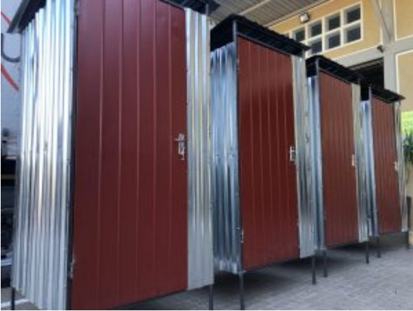
Finished toilet cubicles.
