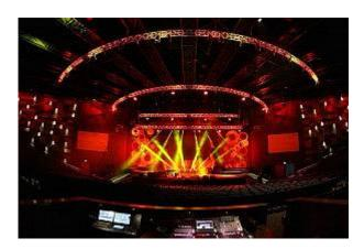
DWR delivered 24 x Robe ROBIN LEDWash 1200s, 12 x ROBIN Pointes and 18 x LEDForce 18 PARs, together with some other generic lighting fixtures, LED truss warmers, a large amount of Prolyte trussing, motors and control; cabling infrastructure, power and data distribution and a grandMA2 lighting console.
