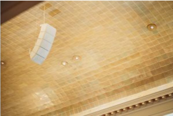
Christ King Parish’s central L-Acoustics A Series array features four A10i Focus enclosures over one A10i Wide
