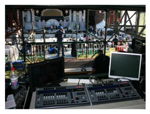
Brisbane Concert Lighting was again the main equipment supplier, supplying all control from LSC Lighting Systems, including Clarity (using 6 DMX universes) with two VX20 wings, five e24 Dimming Systems, five Delta Power Distros and three Delta DMX splitters. The LSC control equipment looked after 44 Martin Moving Lights, 32 LED Par 64s, 32 LED strips and over 72 Fresnels, Pars and Profiles.
