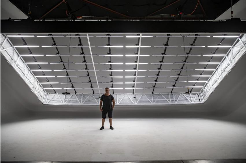
Run wired with data via ArtNet from a laptop, the Titans are controlled via D2 Motion's proprietary software developed by Daniel Miller specifically for the studio and this light box application.
