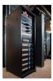
The LSC APS Power Distribution system was selected due to its wide functionality and flexibility. The units are part of the lighting DMX network to allow for central operation of the above-mentioned lighting features; the manager on the day just needs to press a relevant button and the APS takes care of the staggered start-up.
