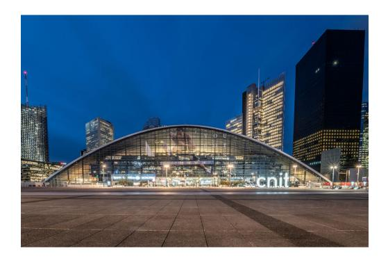
The imposing concrete 'vault' as it is known, is 46 metres high and each side is 218 meters long, forming part of an equilateral triangle. Three glass façades – with convex curves on two sides – each span 206 meters and allow daylight and sun to stream through into the space.
