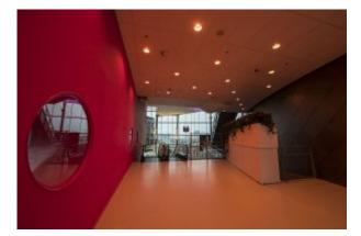
The units are being retro-fitted into the same slots that housed the TivoliVredenburg's old compact fluorescents by the venue's own installation team. They are controlled via DALI, and integrated into the existing KNX building automation system, and can be recalled by Hagar SmartPhone App ... amongst other methods.
