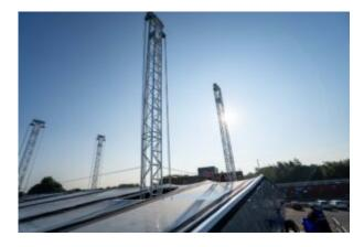
The Space roof gives designers and riggers unprecedented possibilities, with an option to make a rigging point on every square meter. In addition, the roof structure with the Space frames lends itself to walk in, which makes working in this roof safe and easy.
