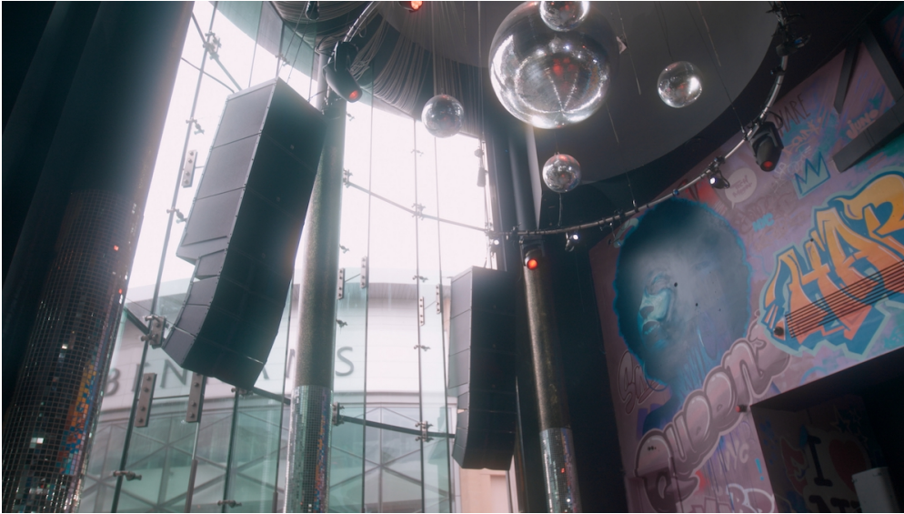
Harlem Club features two flown arrays of L-Acoustics Kara II with SB18.
